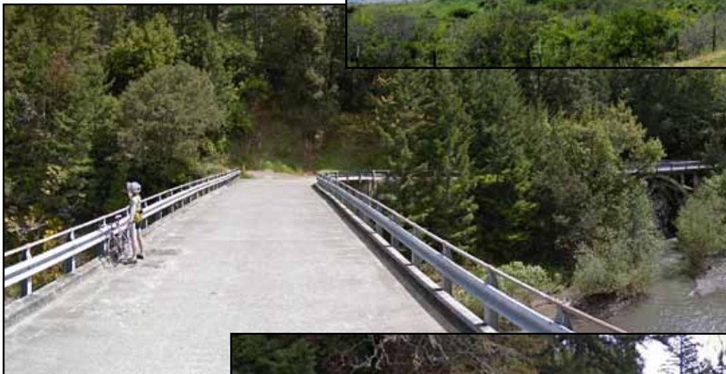
Stage 3: Butler Valley Road crossing the Mad River
